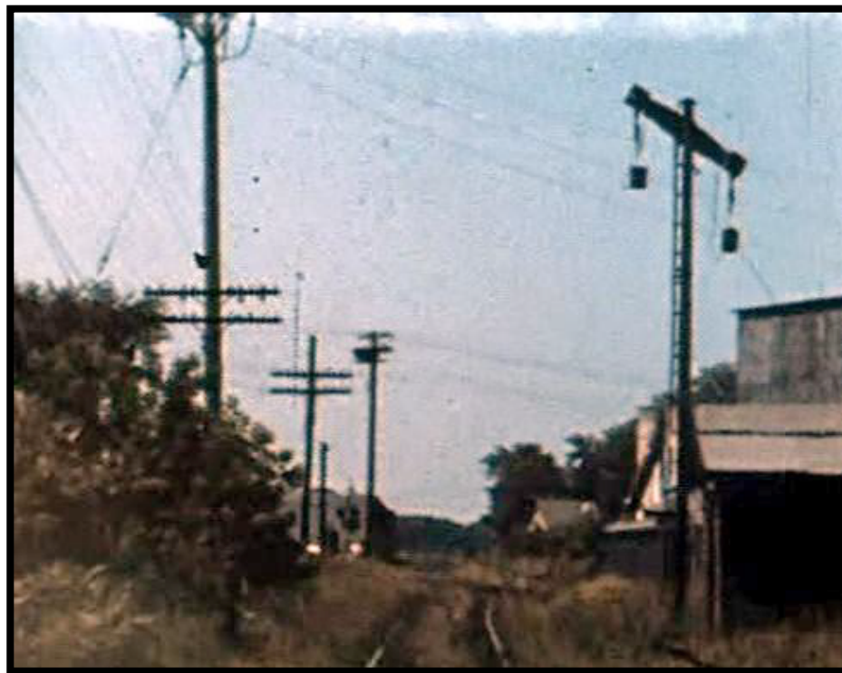
The semaphore in this image is at Schuyler Street in Oswego, NY., also protecting the track crossing at grade of the NYO&W and RW&O successor New York Central. The signal aspect, this image indicates that the O&W is NOT cleared to cross the RW&O/ NYC track. . . . that "Normal" aspect being for the NYC to cross O&W track. Slide image form the Collection of the late OWHRS member "Rusty" Recordon.
