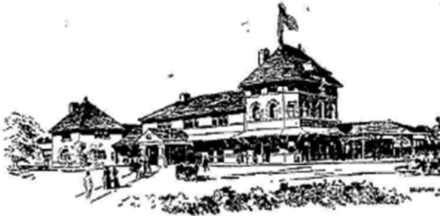
WICKHAM AVENUE STATION, NEW YORK, ONTARIO & WESTERN R. R.
