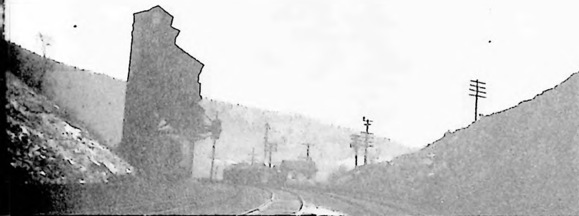
Herb Thieme Looking east at Cadonia in 1947. The coaling tower's days are numbered, but it still sees use as evidenced by the loaded hopper. Note lower quadrant semaphore distant signal for single track at Hawk Mountain Tunnel.
