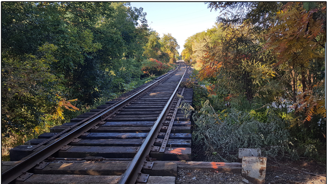
The view in 2019 looking south across the Sauquoit Creek bridge at O&W Milepost 271.84. One of the bridges on my list of responsibilities.
