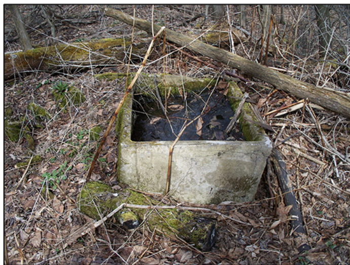
Battery Box on March 27, 2010 (Doug Ellison)
