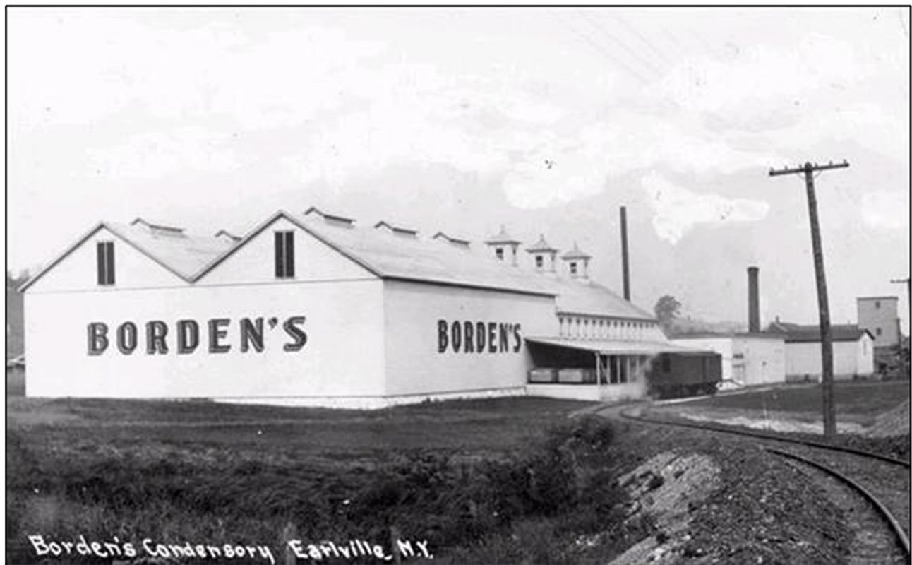
Borden's Earlville, NY on NYO&W "down in the hole" As a kid, I played around here after the building was abandoned. It fell down during the Winter of 1969-1970.
