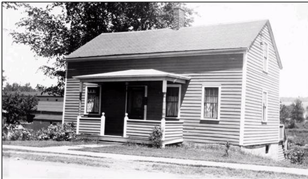
The John A. Ellison home where my father John Jay Ellison was born in 1932. The back yard of this home was where FT 803 would land far into the future in 1955. The coal shed is barely visible to the left. – And yes the middle name is after O&W operator and grandfather Jay Whalen.
